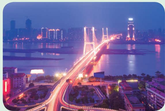
Smart lighting IoT solution powers a smart city
